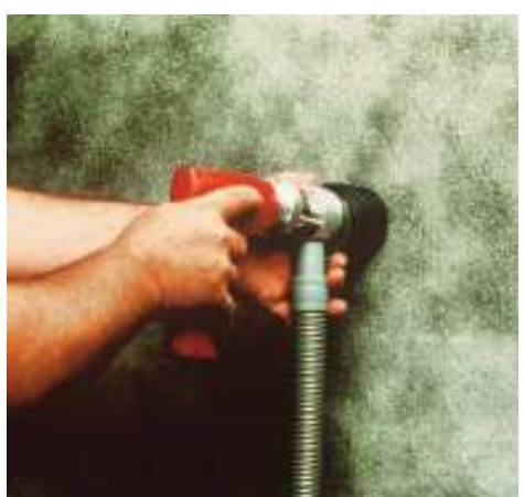
FIGURE 12.19 Needle Gun with HEPA Exhaust Ventilation.
