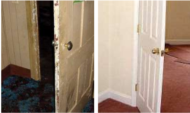
FIGURE 12.4 Pre-and post-abatement interior doors.
