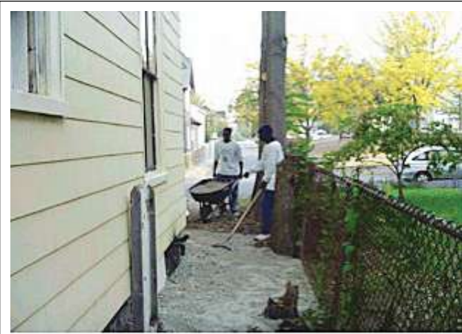
FIGURE 12.23 Preparing to pave high traffic area.
