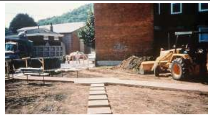
FIGURE 12.22 Replacing resident pathway after soil removal.
