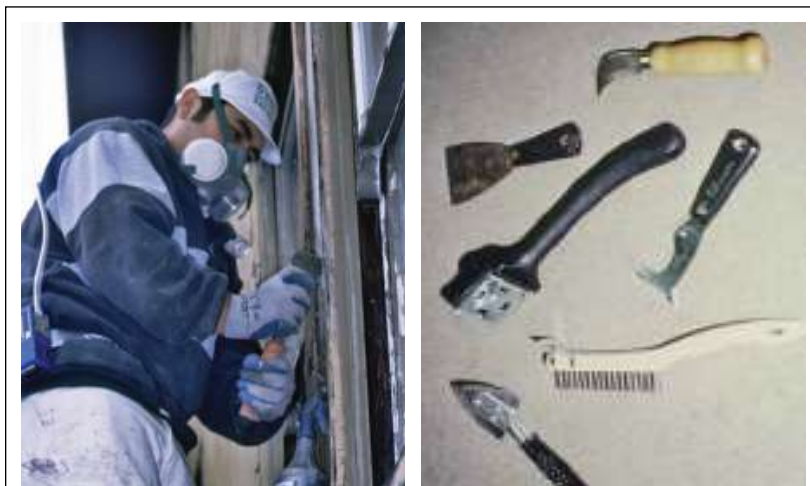
FIGURE 12.16 Wet scraping (left) FIGURE 12.17 Scraping tools (right).
