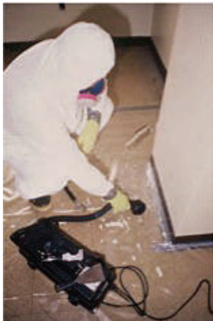
FIGURE 14.8 Vacuuming the floor containment.
