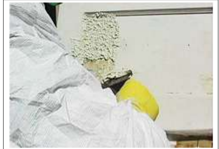
FIGURE 12.20 Workers should wear protective clothing when using chemicals.
