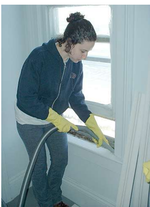
FIGURE 8.17 Pre-cleaning window with HEPA vacuum.
