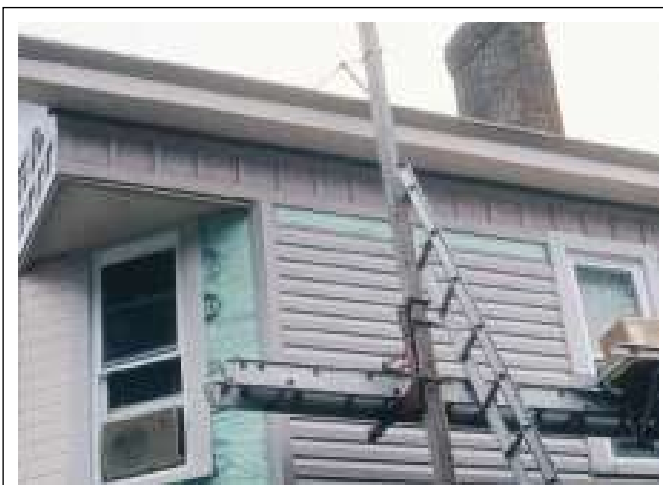
FIGURE 12.6 Installation of replacement siding.
