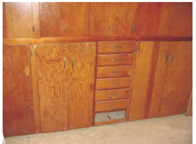
FIGURE 15.10 Surfaces that may have had paint stripped.
