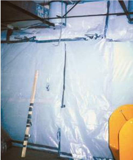
Photo 8: Full containment on large job
