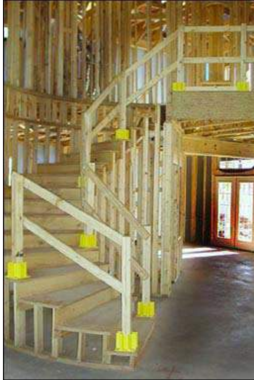
Figure 33 - Wooden guardrail system for a stairway.
