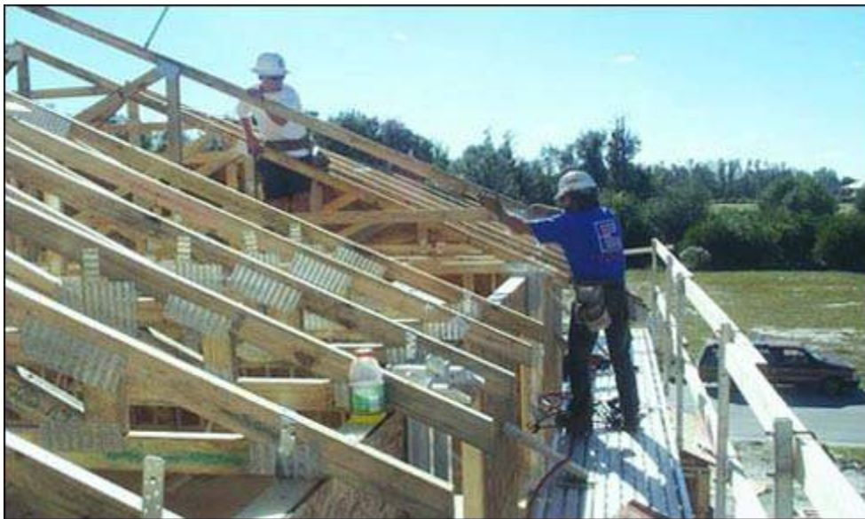
Figure 2 - Workers using an exterior bracket scaffold to install roof trusses.
