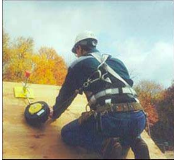
Figure 13 - A worker using a reusable anchor with a retractable lifeline.
