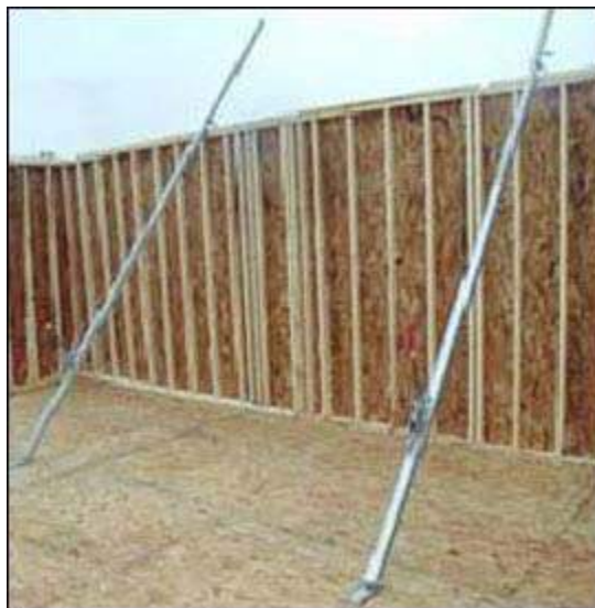
Figure 23 - Framed walls being erected using a jack.
