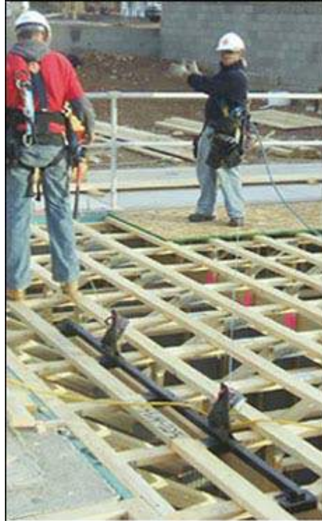
Figure 20 - Workers using a truss bracket anchor while installing a subfloor.
