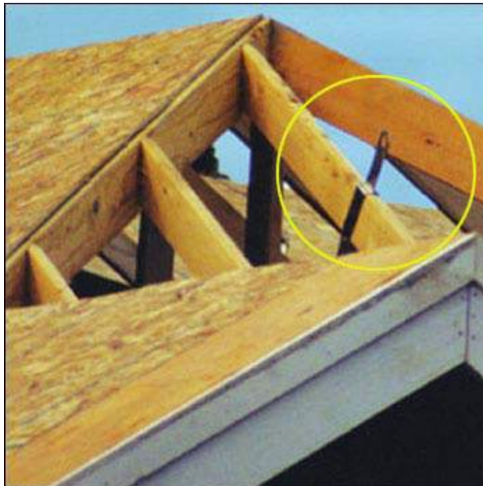
Figure 6 - A bolt-on anchor attached to a rafter.
