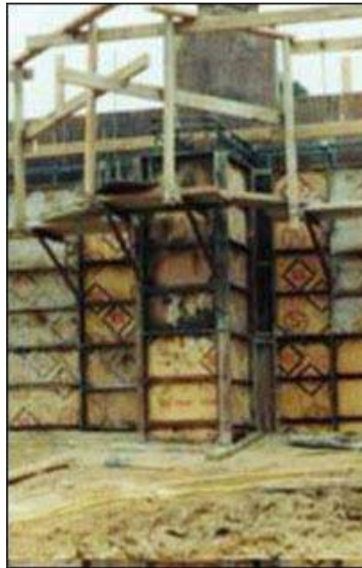
Figure 16 - A bracket-form scaffold attached to formwork.
