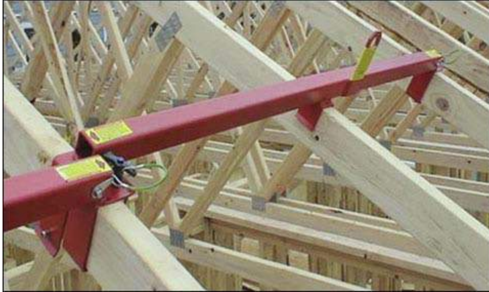
Figure 4 - An example of a spreader attached to roof trusses.
