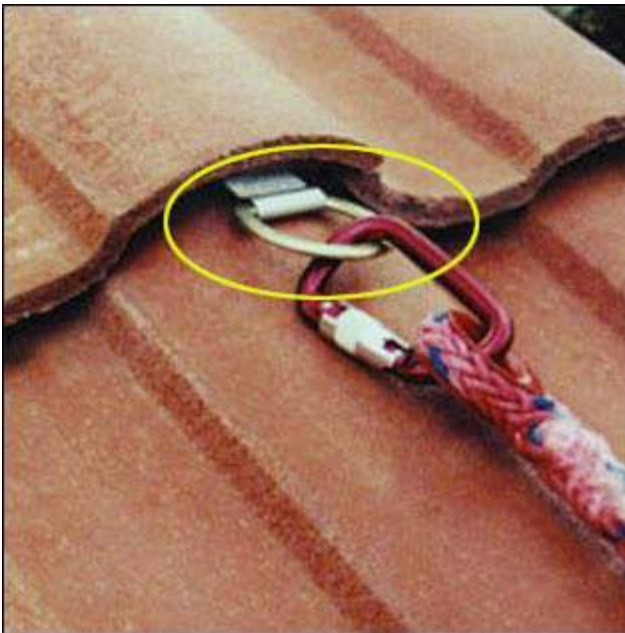
Figures 11 & 12 - Permanent anchors on completed roofs.
