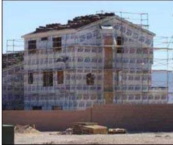
Figure 28 - Welded end frame scaffold.
