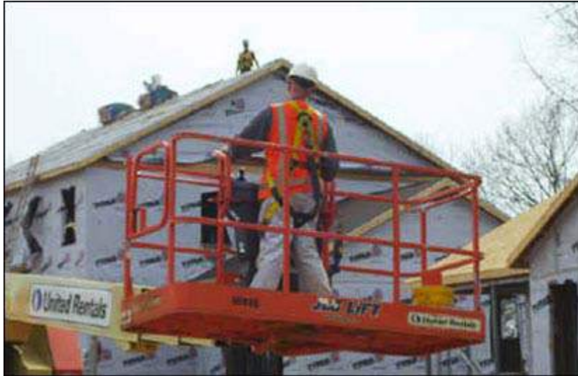
Figure 31 - Worker positioning an aerial lift.
