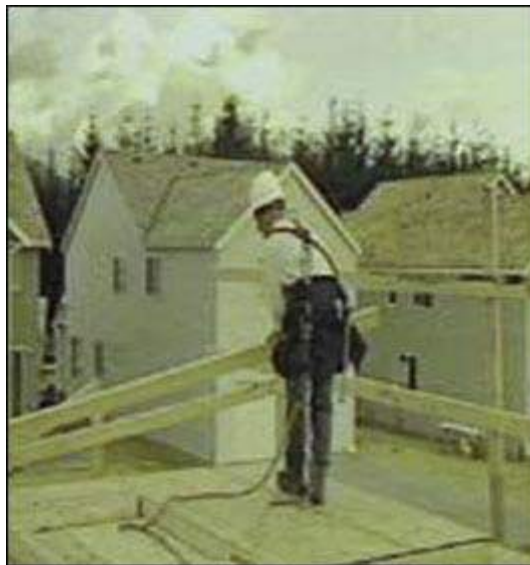
Figure 27 - Worker installing guardrails.
