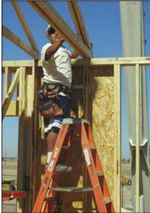
Figure 3 - Platform ladders can be set up inside a structure and used to install roof trusses.
