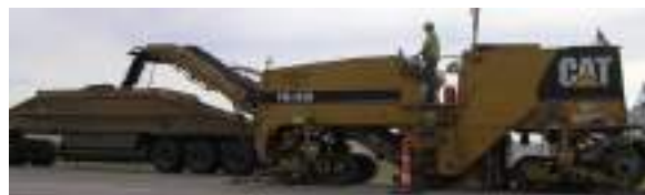
Milling machine milling asphalt road and loading debris into a haul truck.
