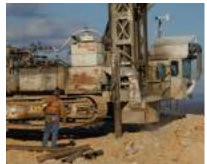
Vehicle-mounted drilling rig using water on the drill bit. The enclosed operator's cab is on the right. Photo courtesy of NIOSH.
