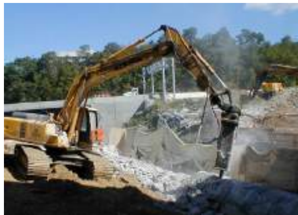
Excavator equipped with an enclosed cab and hoe-ram demolishing a concrete wall.
