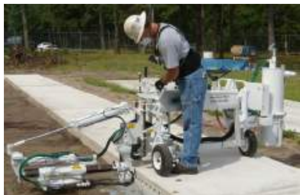
Worker drilling horizontal holes in concrete slab with a dowel drilling rig. The shroud surrounds the drill steel where it enters the concrete and the dust collector is the canister on the right. Worker is wearing respiratory protection.
