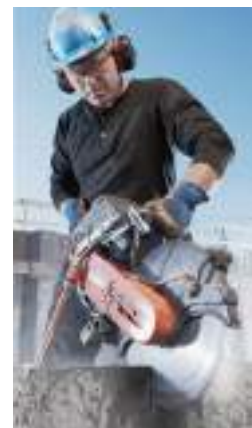
A worker cutting a concrete block using a handheld masonry saw with an integrated water delivery system.
