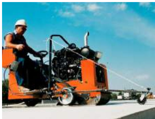
Worker cutting a groove in concrete roadway with drivable saw using integrated water delivery system.
