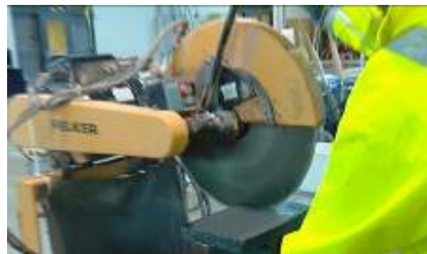
Worker cutting masonry block on a stationary masonry saw equipped with integrated water delivery system that continuously feeds water to the blade. Note water supply hose attached to top of shroud around blade.
