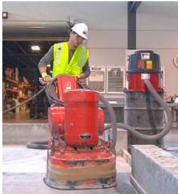
Worker milling granite floor indoors with milling machine and dust collection system (background).
