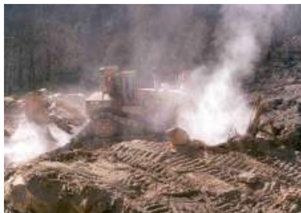
Earthmoving using a dozer equipped with enclosed operator cab. Photo courtesy of NIOSH.
